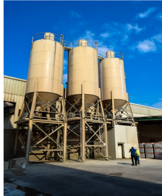
Dedicated Silo for Solidia Cement
