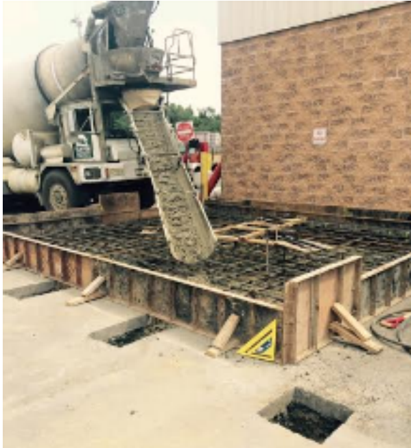
Concrete Pad for CO 2 Storage Tank
